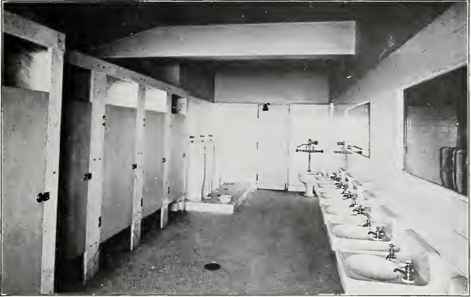
FIG. 138.—Toilet room, Post Hospital, Rockwell Field, Calif.
